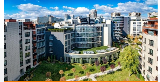
Green Roofs, Parking Lots, Pedestrian Area, and Special Facilities
